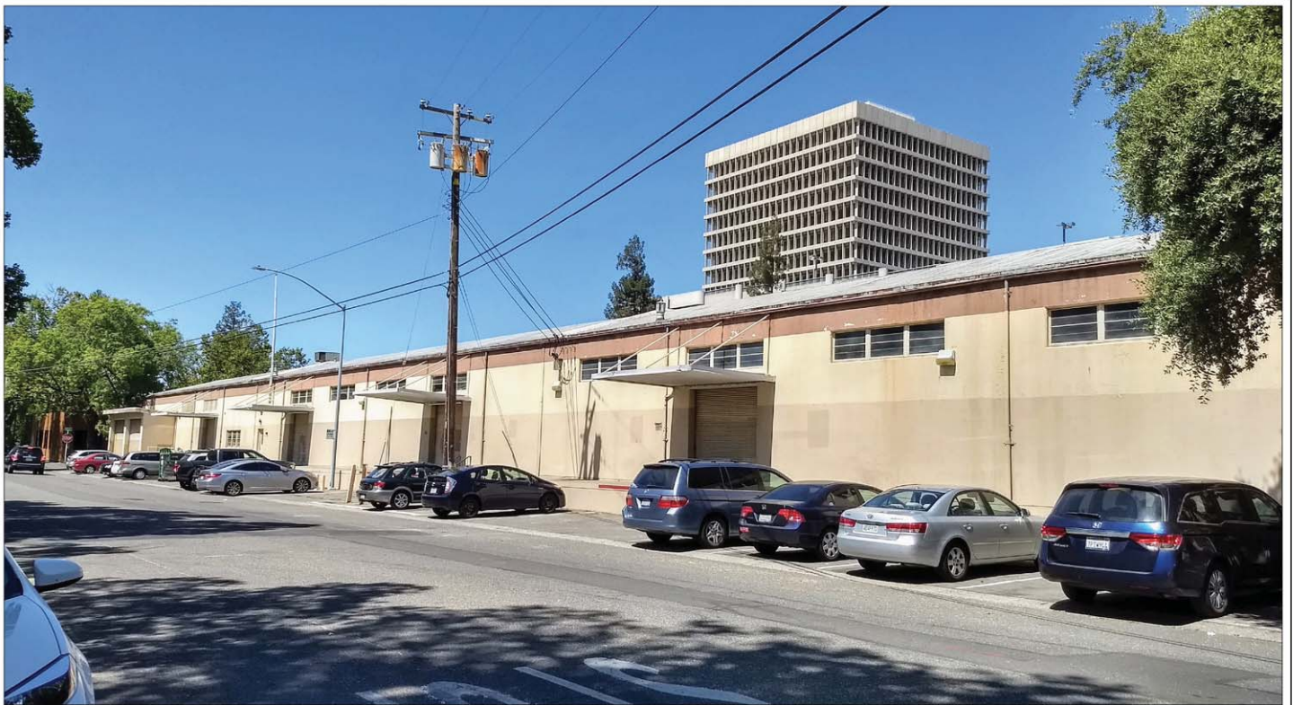
DGS warehouse at 805 R Street, view from 9th and R Street.
